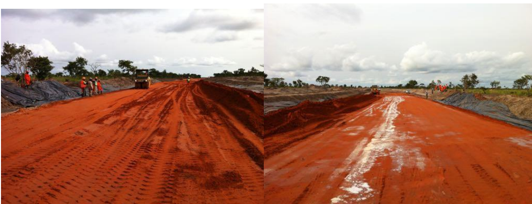
*Leveling and profiling of the surface
