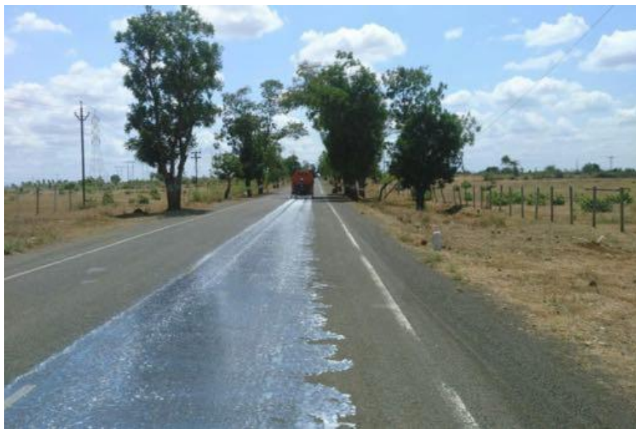
Sealing irrigation on asphalt mix. India
