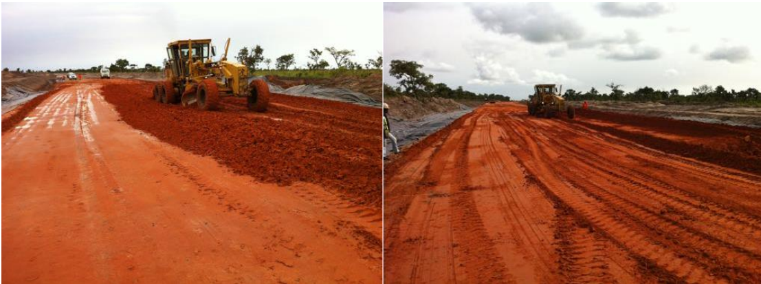
*Preparation of the material to be stabilized
