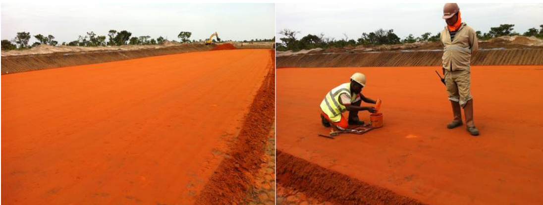
*Compaction required in project.
