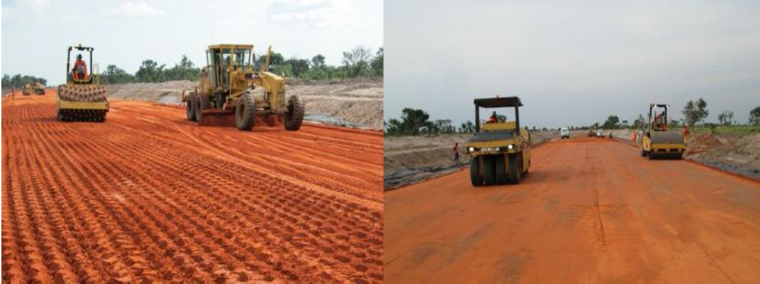
*Roller compaction
