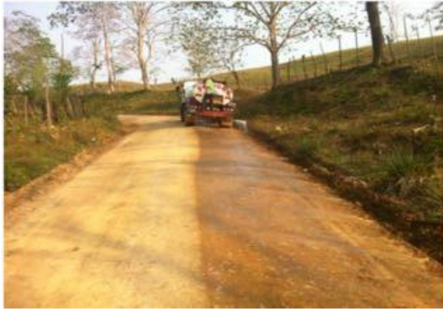
Sealing irrigation on compacted track. San Pedro de Urabá (Colombia)
